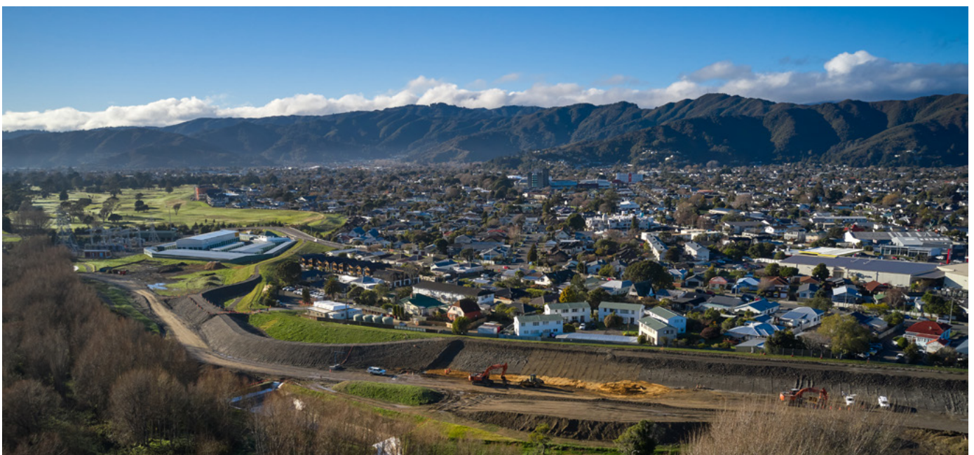
Mills Street stop bank, Riverlink Project. Greater Wellington Regional Council
